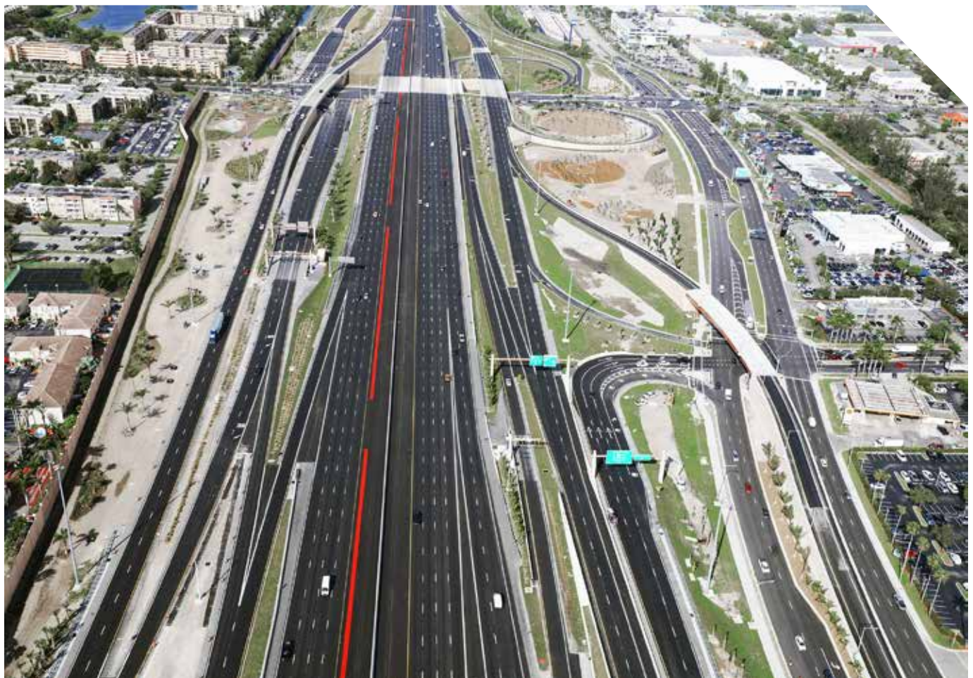
SR 836 Interchange Modifications at 87th Avenue, looking westbound along SR 836 at NW 82nd Avenue.
