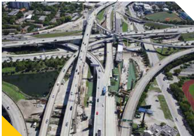
Project 83611 – SR 836/I-95 Interchange Improvements
