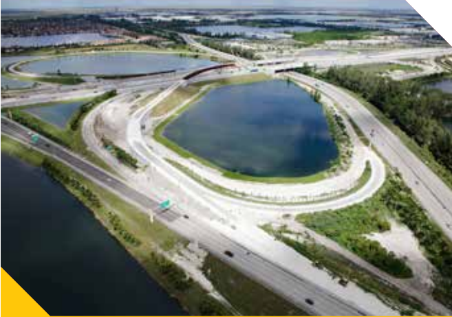
Project 83634 – SR 836 New HEFT Ramp Connections
